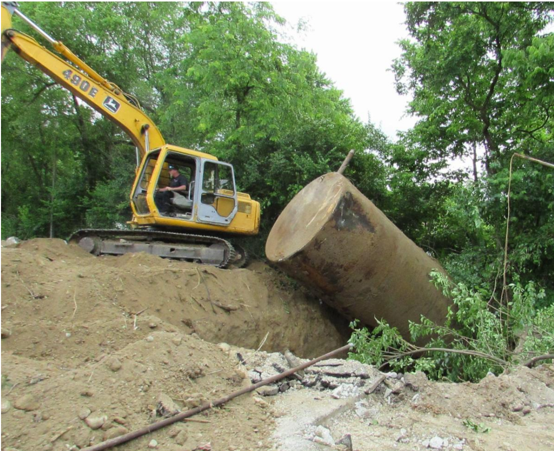
Demolition and tank removal, former Omega Oil site, 2036 N. Gettysburg Ave.
