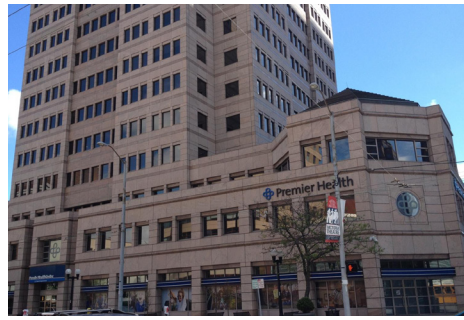
PREMIER HEALTH CENTER
