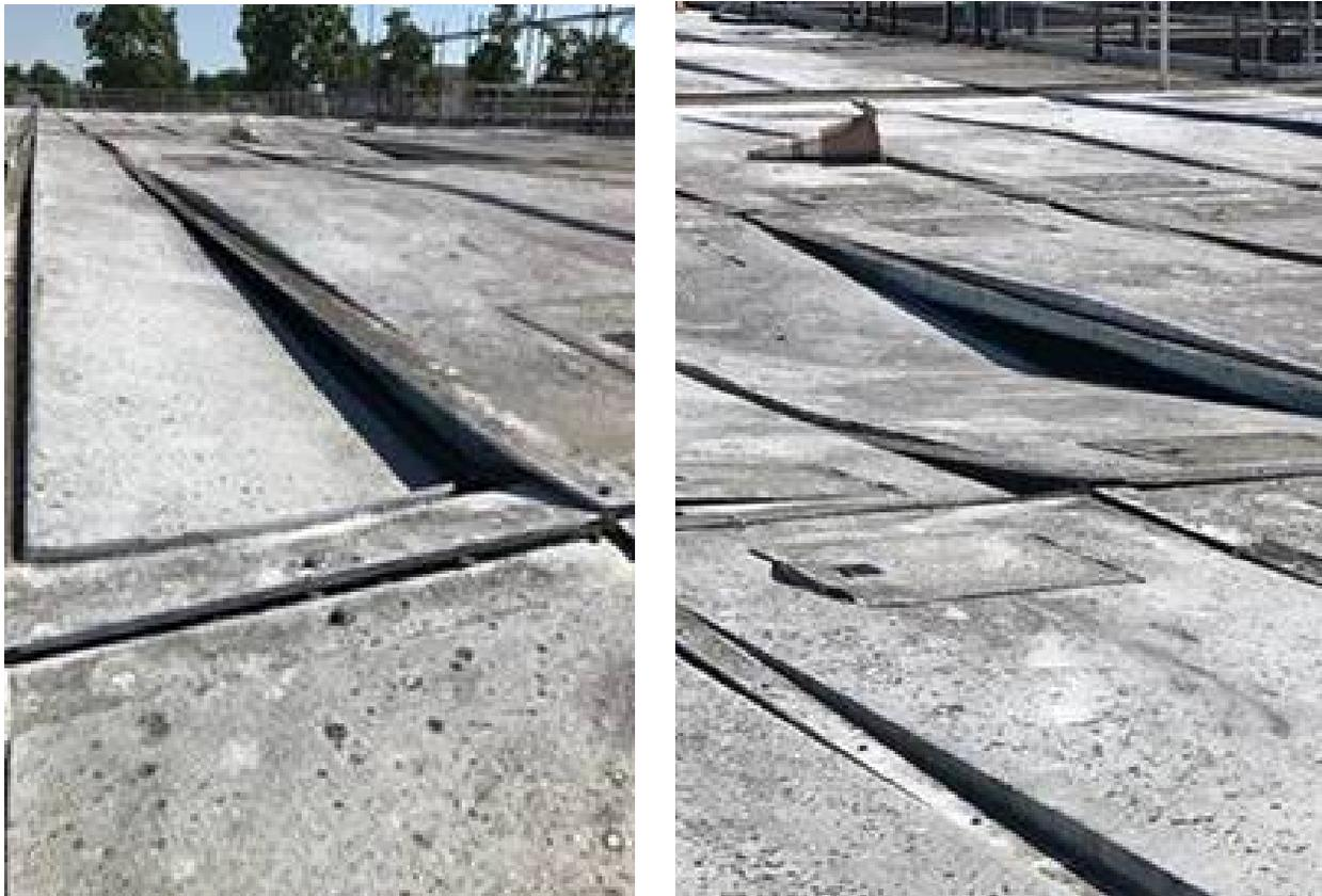
**Figure 3. Photos of the deteriorated and broken odor covers**
