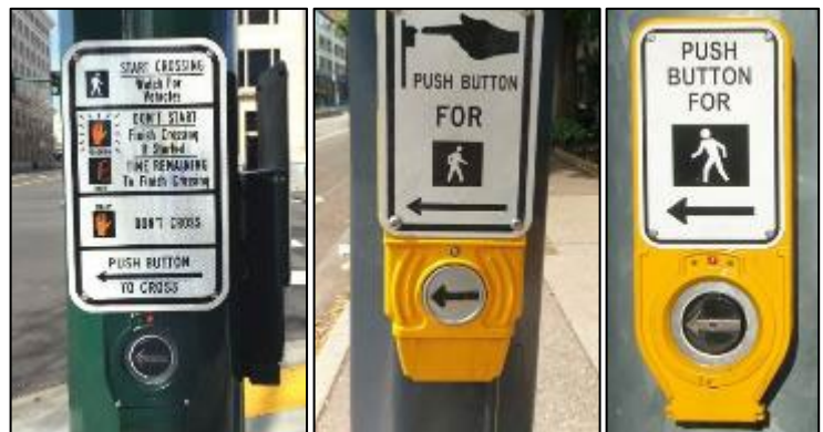
Examples of various options for updated pushbuttons with compliant tactile directional arrows and updated signage.
