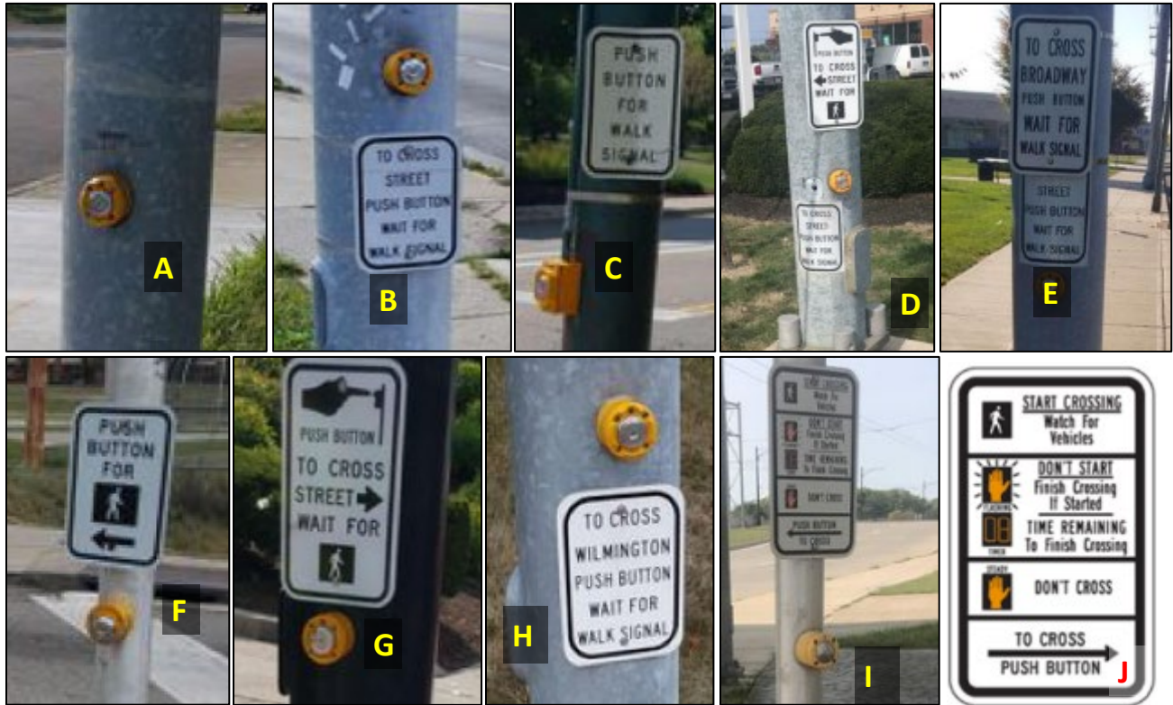
Examples of various signs provided at pedestrian pushbuttons, including (A) no signage, (B) and (C) generic text instructions with no identification of street crossing controlled, (D) and (E) multiple signs for the same pushbutton with different orientation/information, (F) and (G) signs that provide text instruction and an arrow indicating the crossing controlled, (H) text only sign that includes description of crossing controlled, (I) current standard sign with detailed text instructions with directional arrow indicating the crossing controlled and pictures adjacent to the instructions, and (J) enlargement of current standard sign.
