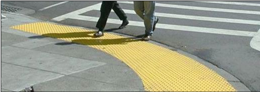
Diagonal blended transition. Note the level transition from the street crossing to the PAR.
