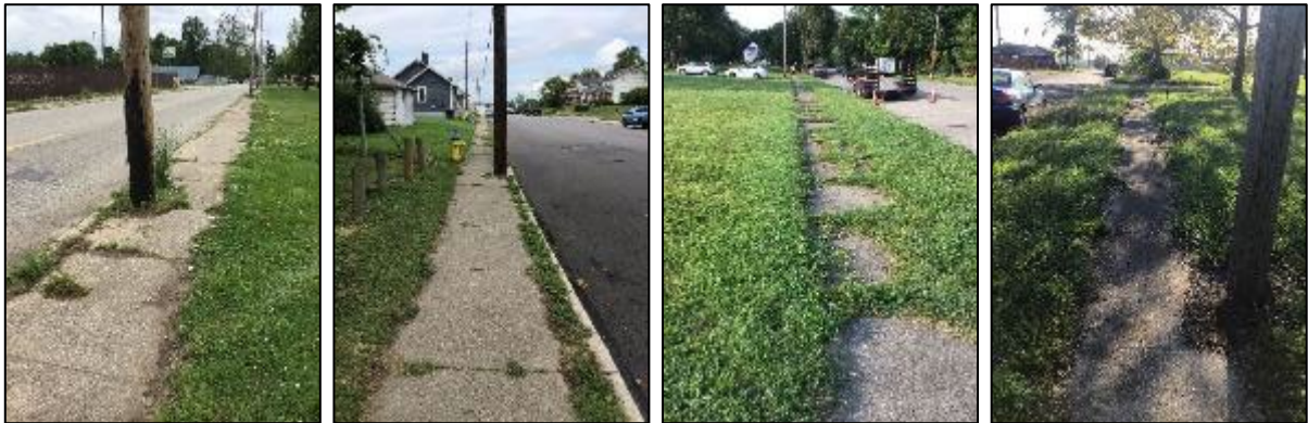
Examples of obstructions of the PAR that reduces the width to less than 48".
