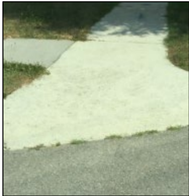
Curb ramps lacking DWs as required or which have low contrast.
