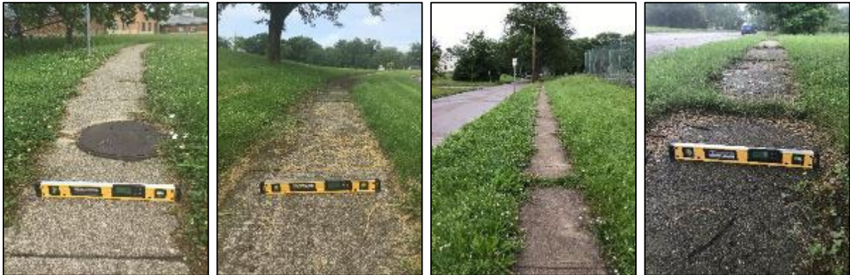
Examples of sidewalk that is less than 60" in width (24" level for reference) and often also in poor condition.
