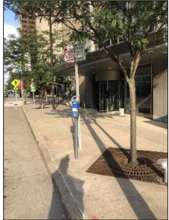
Accessible space located at the end of the parking zone that provides a loading zone and long travel distance from the space to the corner curb ramp.
