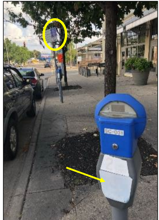
Two accessible parking spaces in area with wide sidewalks, both with faded ISA, no curb ramp or access aisle, and not at end of the block. Note sign delineating accessible parking zone with non-accessible space beyond sign.
