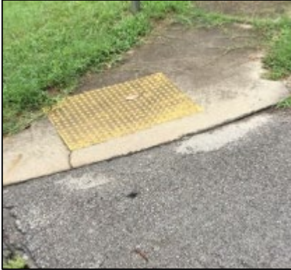
DWs that are oriented poorly and are not 24" depth in entire direction of pedestrian movement.
