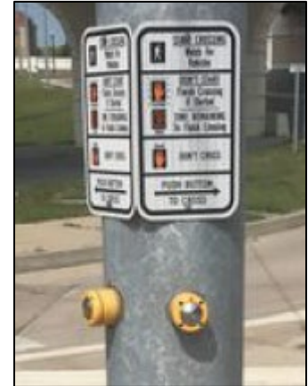
Example of 2 pushbuttons on the same pole.
