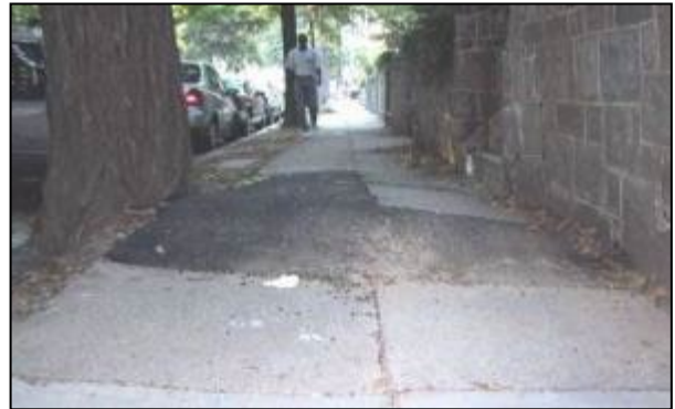
Temporary patching for large displacements
