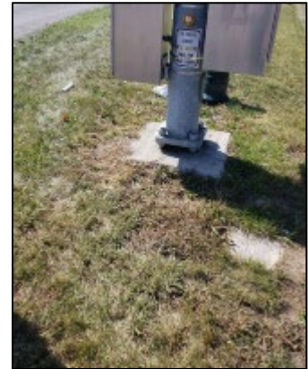
Pushbutton that is not located on an accessible route.
