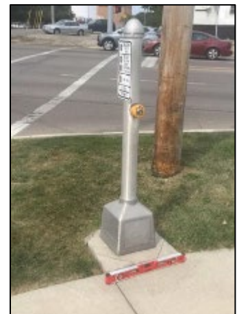
Example of pushbutton with face not parallel to the crosswalk.
