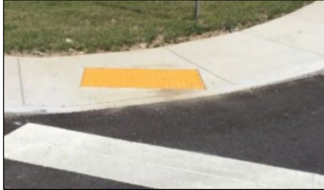
DWs that are oriented poorly and are not 24" depth in entire direction of pedestrian movement.
