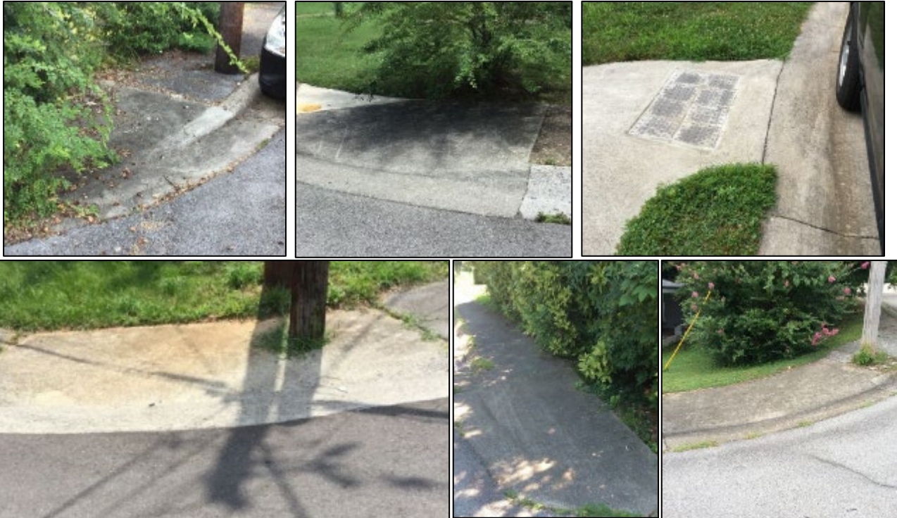
Examples of curb ramps with obstructions at turning spaces, on the ramp, or immediately adjacent to either.
