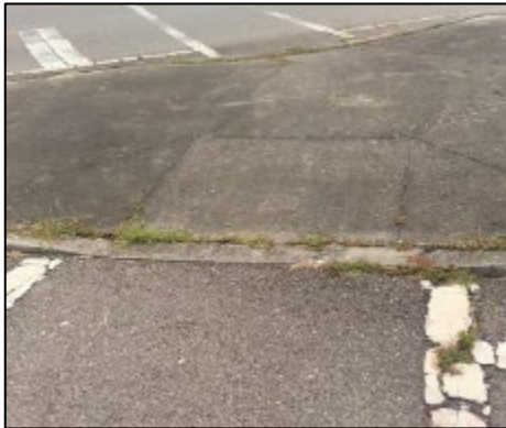
Curb ramps lacking DWs as required or which have low contrast.
