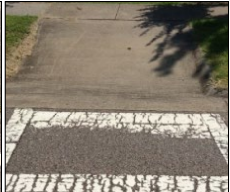
DWs that are oriented poorly and are not 24" depth in entire direction of pedestrian movement.
