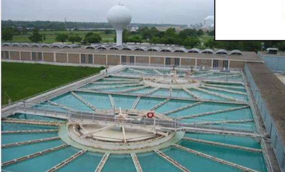
Miami Water Treatment Plant
