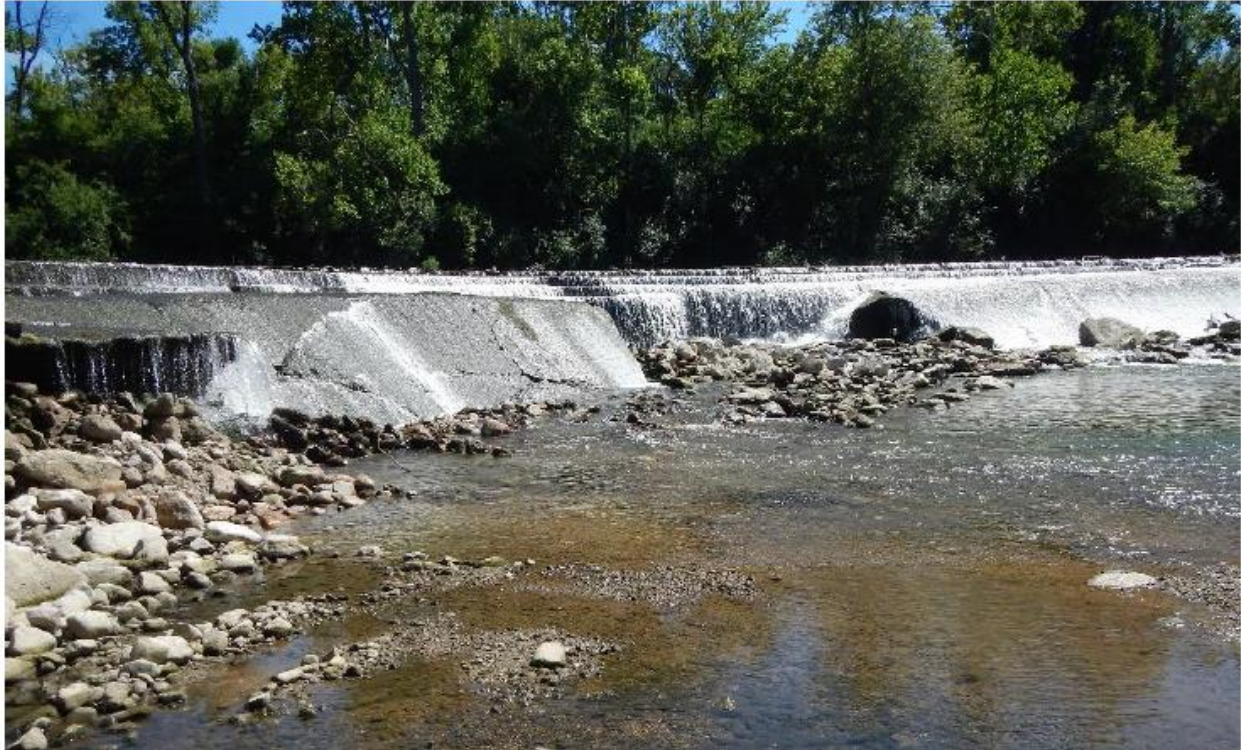
Figure 3. Photo of existing dam, showing broken portion of dam.
