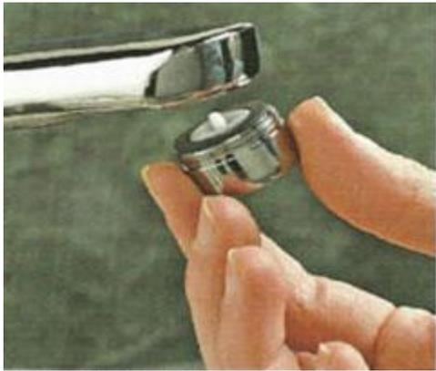
Step 4. Reassemble the aerator, screw it back onto the faucet and hand-tighten. If any parts are cracked or broken, replace them. If the washer has hardened it should be replaced.
