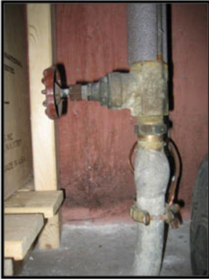
Lead service lines can be connected to the residential plumbing using solder and have a characteristic solder "bulb" at the end, a compression fitting, or other connector made of galvanized iron or brass/bronze.
