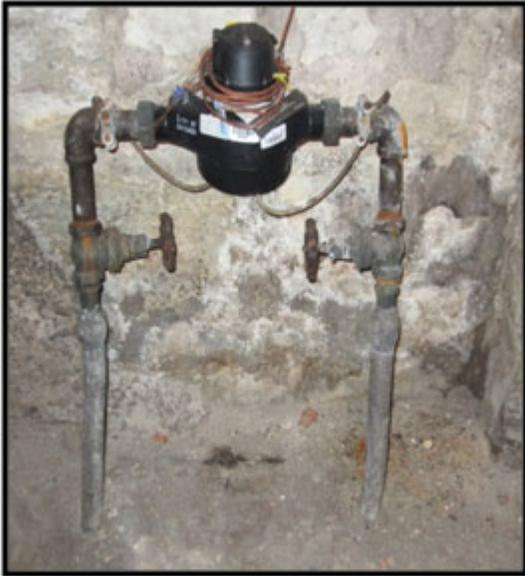
Lead service lines often end just inside the front or side wall of the home, but may extend further into the building as shown, where the lead service line comes out of the basement floor to the water meter and then back into the floor, continuing further into the building.
