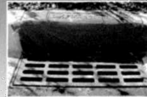
Combination inlet with magnetic rear guard attachment
